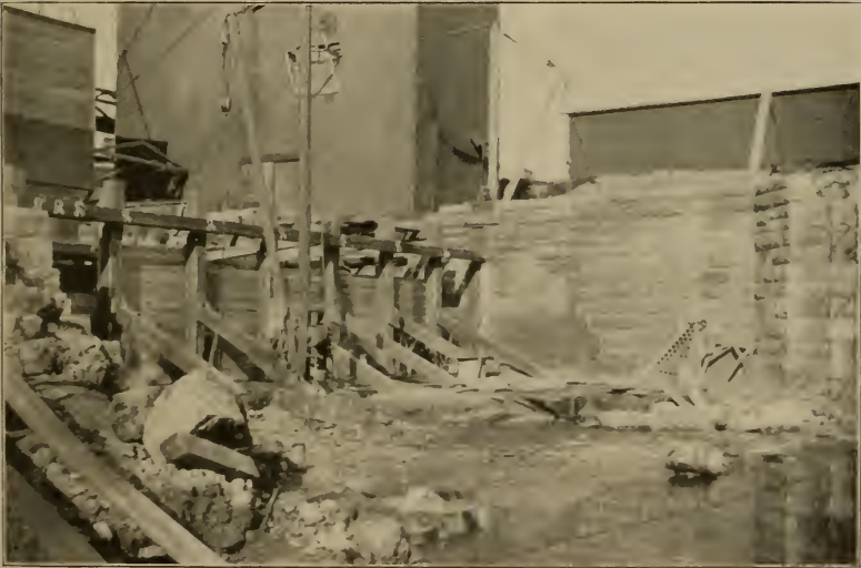
HEAD GATES—ROCKFORD GENERAL ELECTRIC CO.
